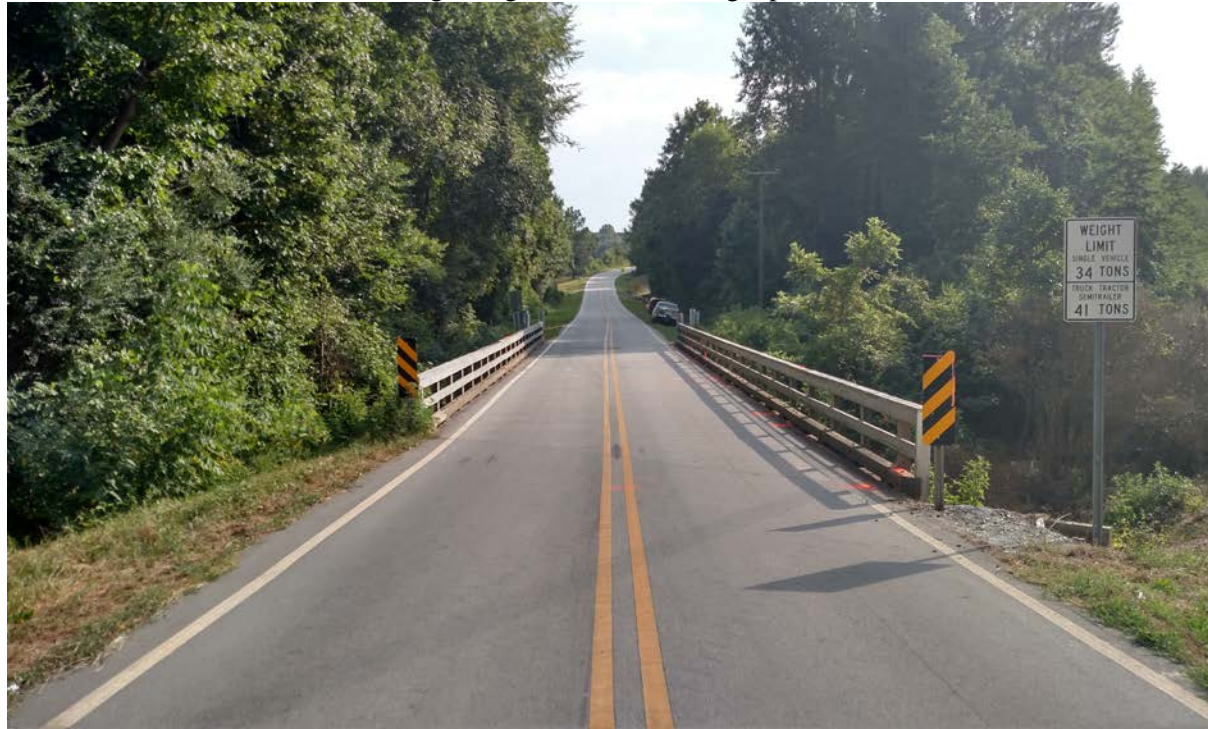
View of Existing Bridge No. 175 Looking Upstation
