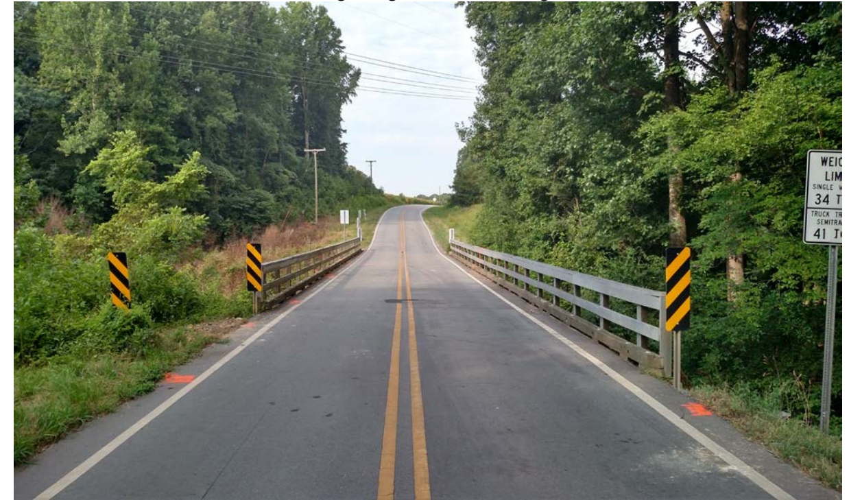
View of Existing Bridge No. 175 Looking Downstation
