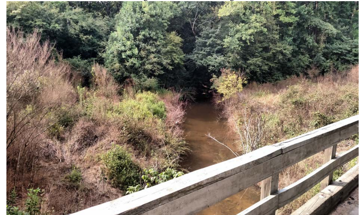
View Looking Downstream from Bridge No. 175
